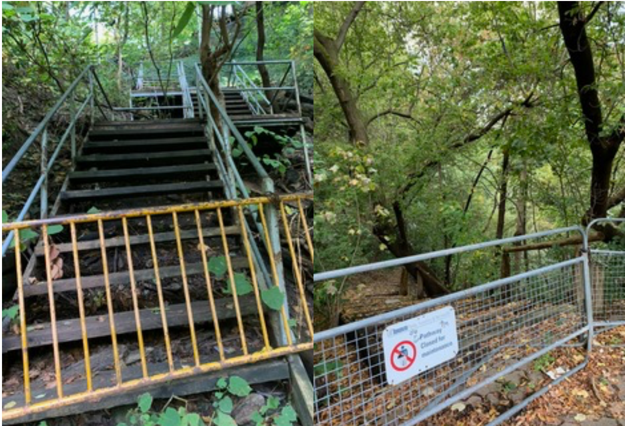
Deteriorated accesses to Yellow Creek / Vale of Avoca at Heath St E and on the north side of St Clair
